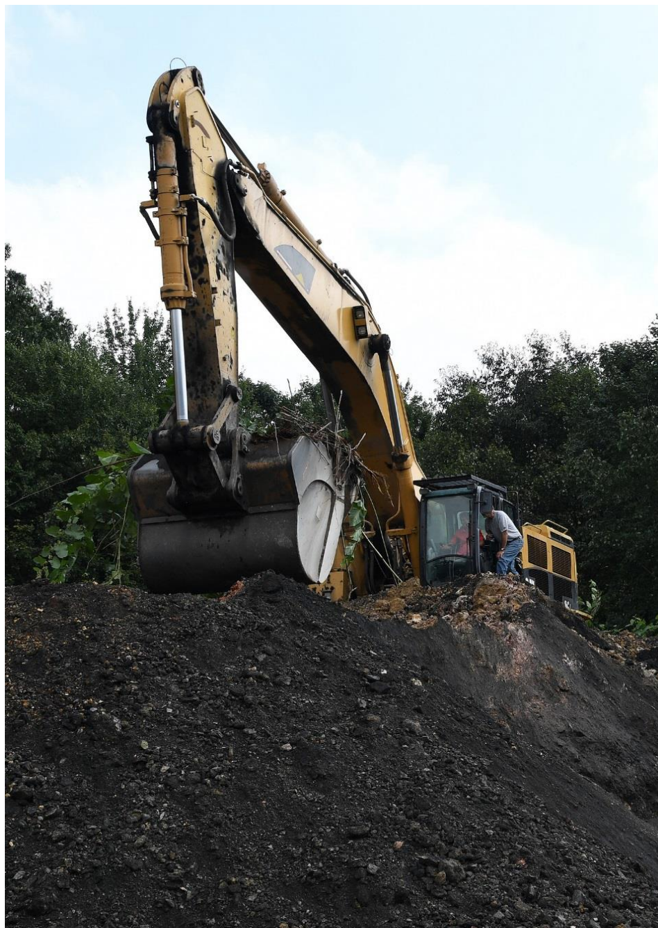
Excavator working at the Ehrenfeld Abandoned Mine Reclamation Project Photo Credit: U.S. Dept. of the Interior
