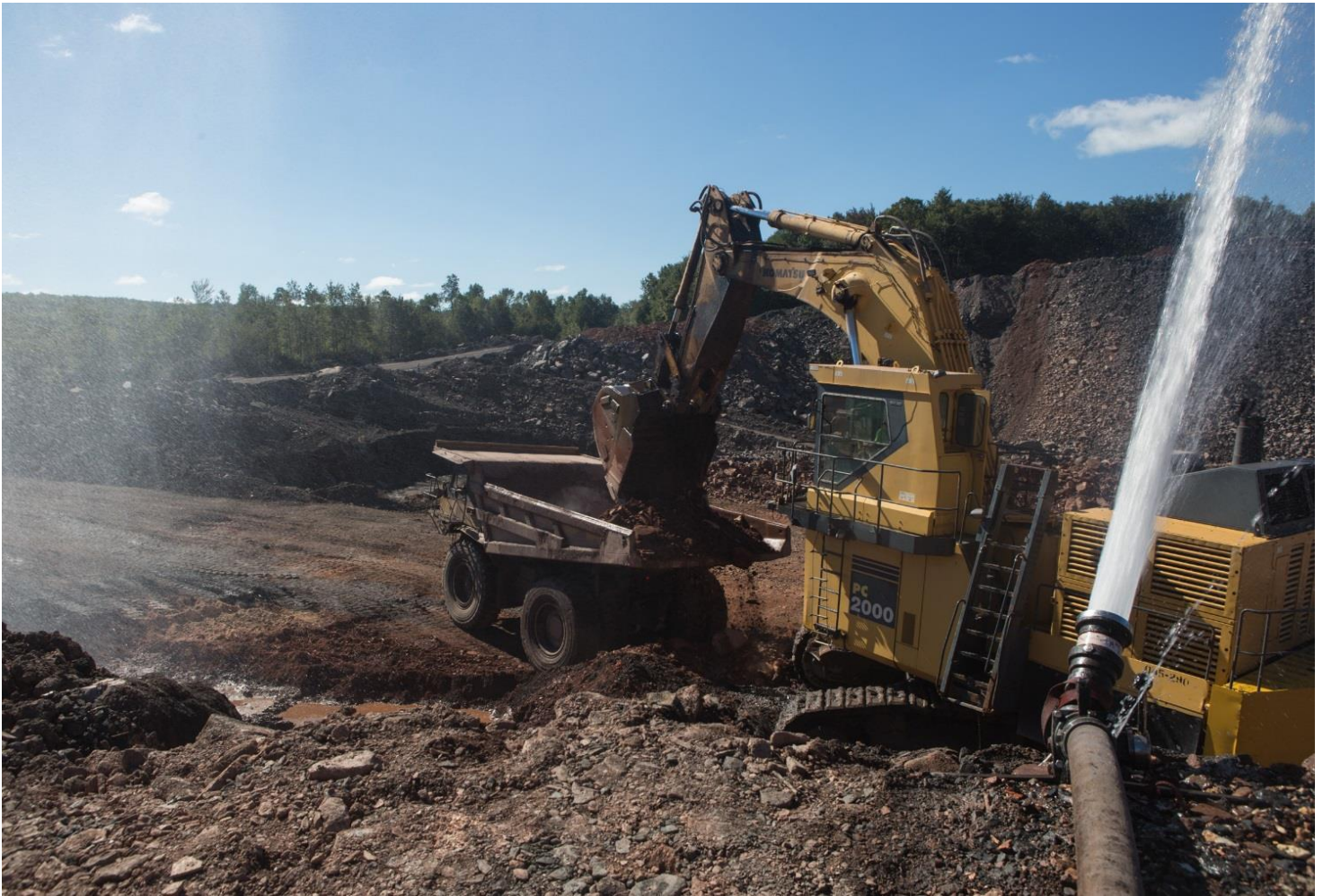
Powderly Mine Underground Fire Site – Photo Credit: Pennsylvania Department of Environmental Protection
